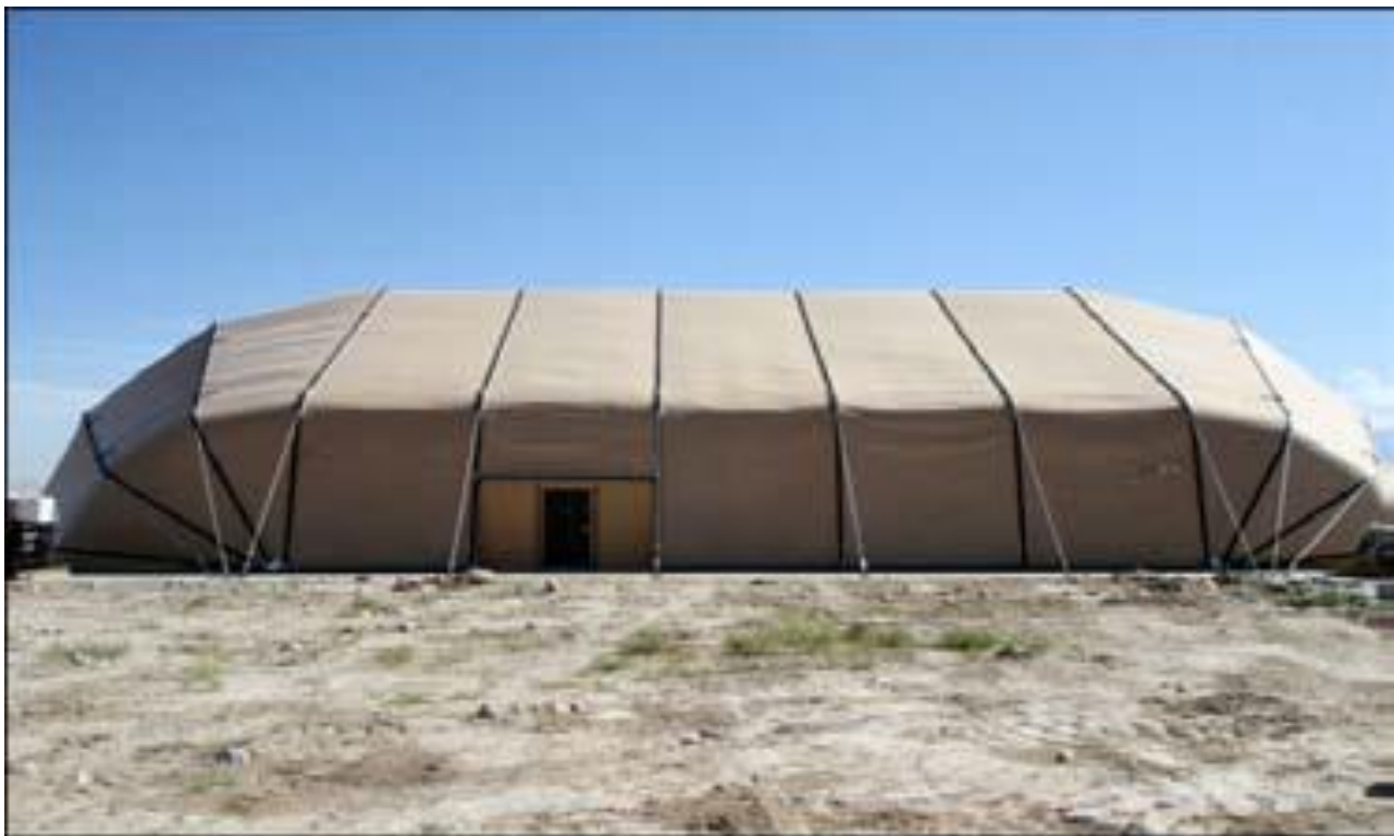
Figure 5: LAMS, large shelter used to house aircrafts [19]
